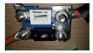
The fuse is located on the space betwee left and right stern cabins on starboard wall. The anchor windlass fuse is 100 amps. You can replace the fuse if it is burn out.
